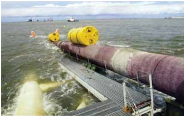
Shallow water pipelaying
