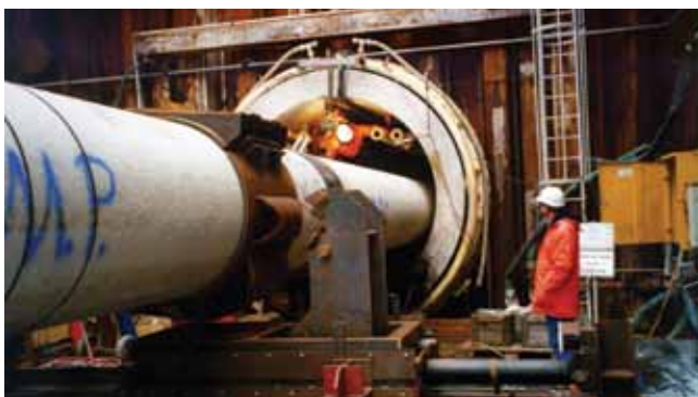
Pipeline installation at landfall tunnel
