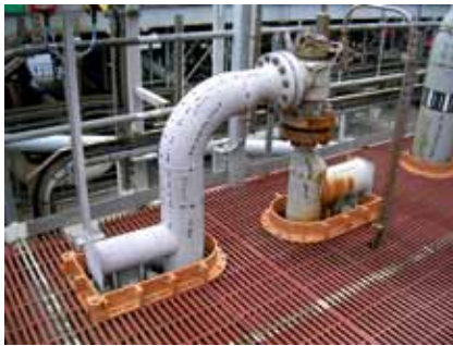
Water flood piping of FPSO Bonga
